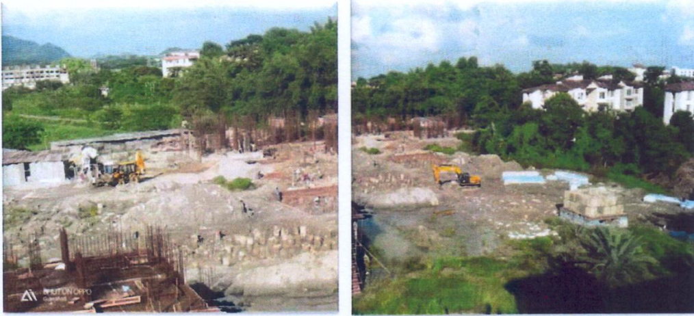
F - TYPE FOUNDATION WORKS. PILE TEST [Signature]
